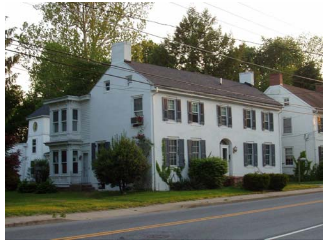
L.D. Caulk House, Circa 1810 228 E. Camden-Wyoming Avenue
