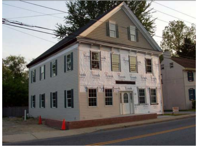
Odd Fellows Building Circa 1850 240 E. Camden-Wyoming Avenue
